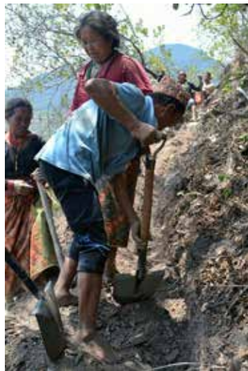
Digging the new trench on the steep mountainside.
